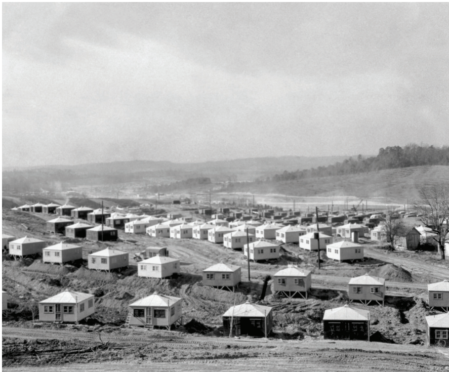
Homes under construction in Oak Ridge, Tennessee, circa 1945.
